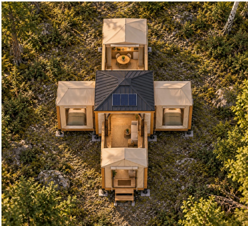
Completed cabin appearance
